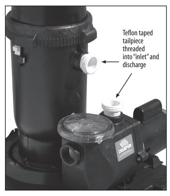
1. Install threaded union adapters on inlet to filter and discharge (top) of pump, using Teflon tape supplied. Use four wraps of the Teflon tape on adapter for proper seal.
