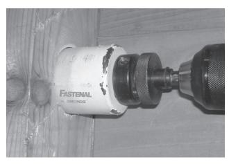
2. Mark where the drain is to be positioned and using a 2" hole saw, drill a hole through the spa wall.
