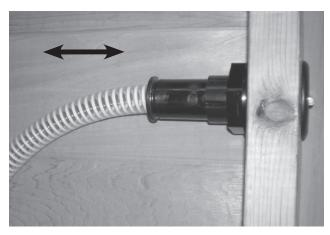
1. Find a place around the lower perimeter of the spa where the drain can be installed. The hose on the back must be allowed to travel several inches back and forth freely.
