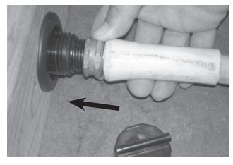
9. To disconnect the hose, push the hose inward approximately  $\frac{1}{2}$ " to shut the water flow off. Unthread the hose.
