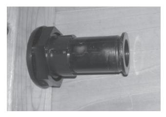
3. Slide the body of the spa drain through the hole and secure with the nut. Silicone can be added to the threads to prevent the nut from backing off.
