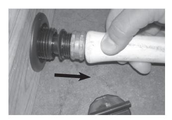
8. Pull the hose outward to allow water to flow. Push inward to shut water flow off.
