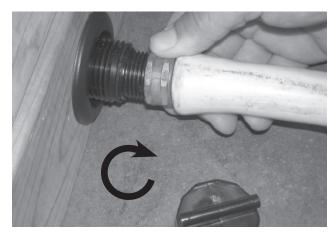
7. Thread hose onto the spa drain.
