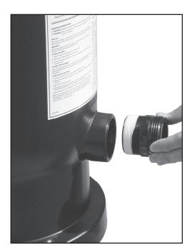
5. Wrap 3 or 4 turns of Teflon tape (provided) on 2" x 1  $1\!\!\!/ 2$ " MPT union fitting and install into "outlet" of filter.
