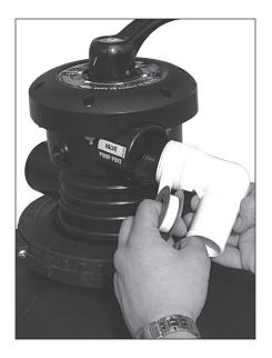
**8.** Apply Teflon tape to smooth 90° hose adapter threads (4 wraps) and thread into valve pump port.
